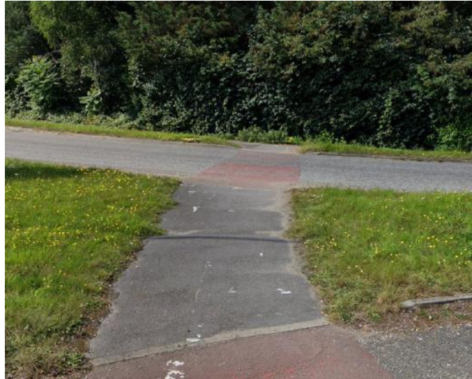
Photograph 20: Ashley Heath Roundabout Crossing Facility
