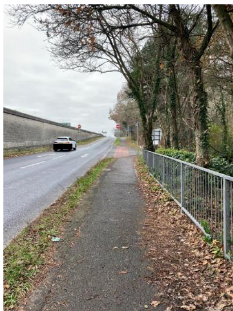
Photograph 6: Folly Farm Lane Crossing Facility
