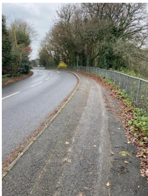
Photograph 5: B3081 Shared Foot/Cycleway
