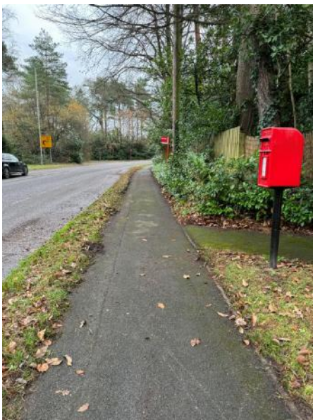
Photograph 21: Horton Road Footway
