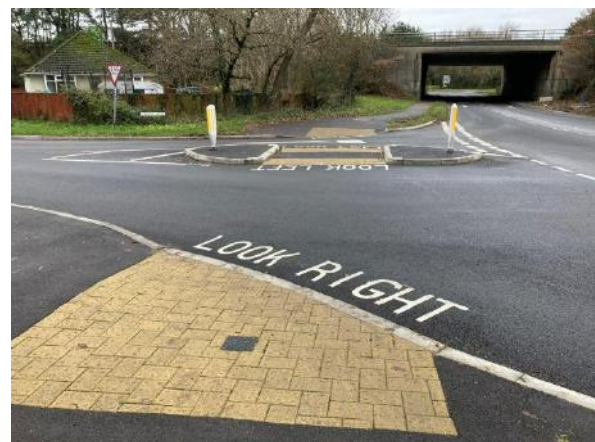
Photograph 4: Hurn Lane Crossing Facility
