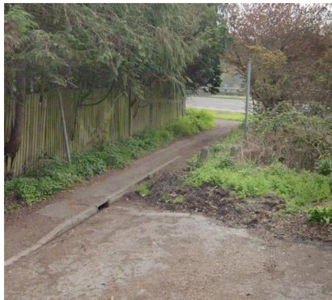
Photograph 22: Horton Road/A31 Footway Connection
