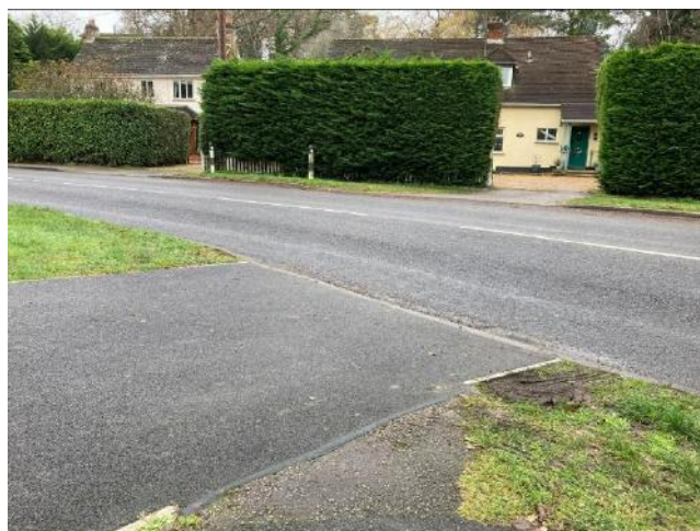
Photograph 12: Hurn Lane Dropped Kerbs Infrastructure
