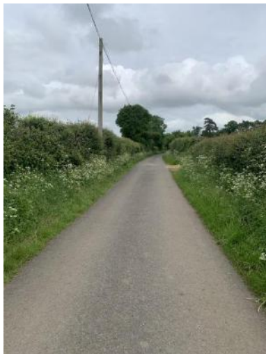
Photograph 21: Existing Conditions along Lomer Lane
