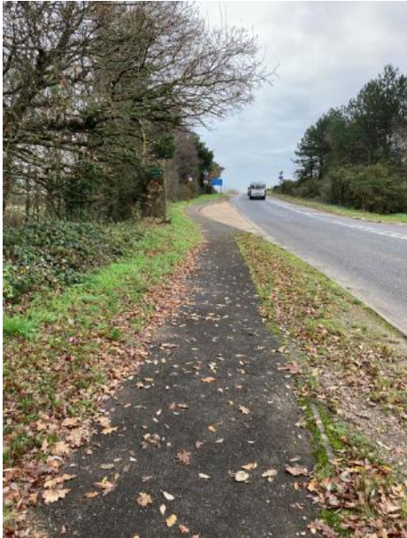
Photograph 1: Verwood Road (B3081) Northeastern Footway
