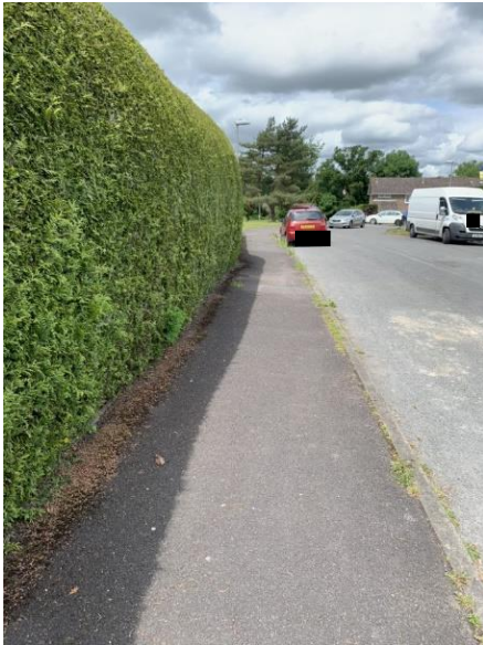
Photograph 15: Footway along Windsor Way
