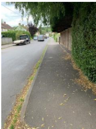
Photograph 3: Footway along Ringwood Road
