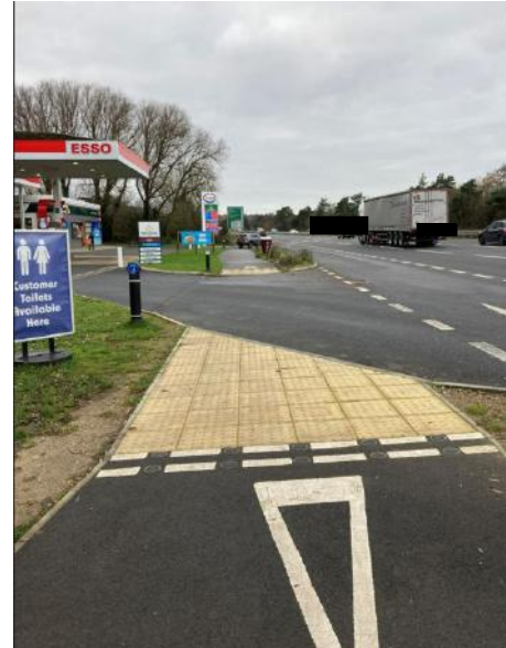
Photograph 16: Shared Foot/Cycleway Infrastructure
