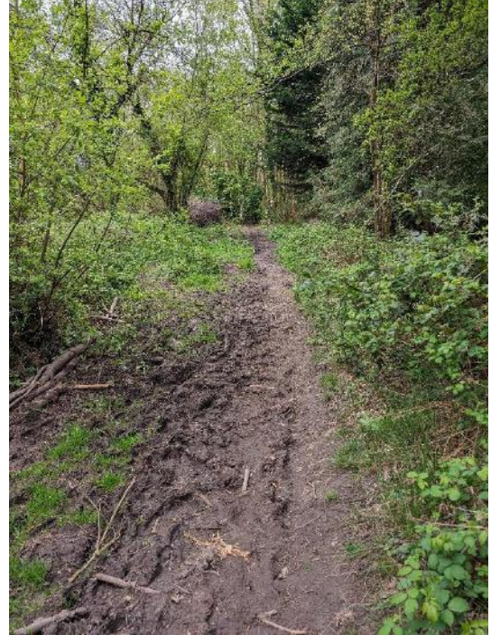
Photograph 32: Existing Conditions along Footpath E34/4
