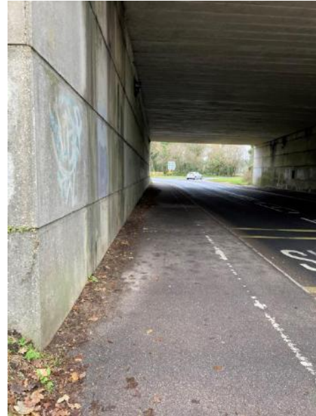
Photograph 2: Verwood Road (B3081) Southern Footway
