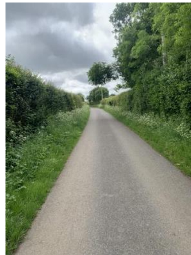
Photograph 22: Existing Conditions along Lomer Lane
