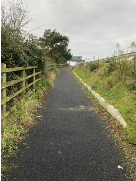
Photograph 15: Footway along A31
