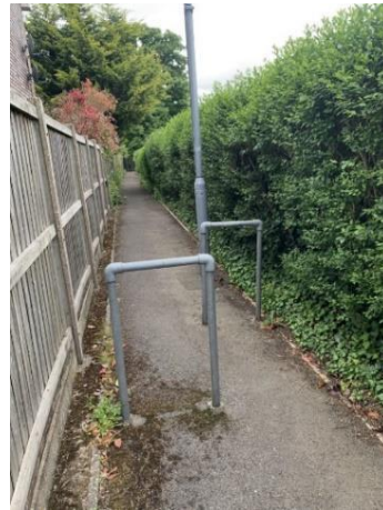
Photograph 8: Footpath at Route 'I' Ringwood Road End
